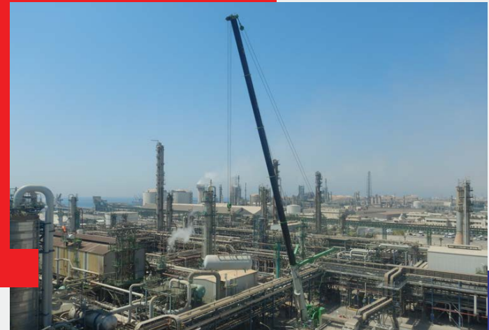
Qatar Petrochemical Projects
