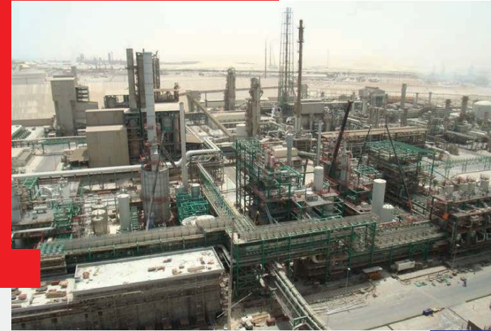
QATAR FERTILIZER COMPANY (QAFCO) MELAMINE & UREA REVAMP PROJECT @ MESAIEED
